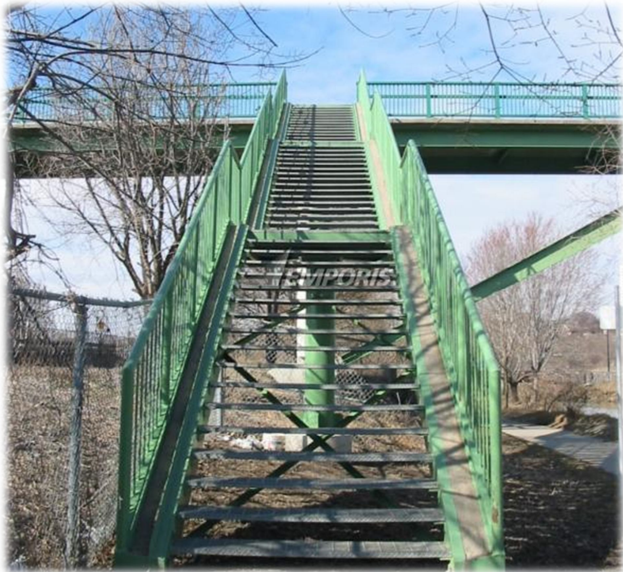
Figure 8: Pedestrian Staircase with Bicycle Runner Rails.
